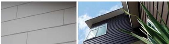
Hardboard plank and siding. (Fiber cement)
