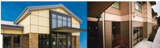
Examples of use of Hardboard plank and siding. (Fibre cement)
